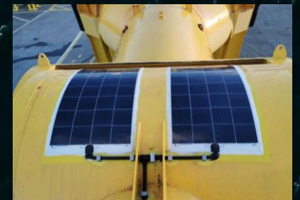
Showing solar panels at hinge & forward wave channel.
